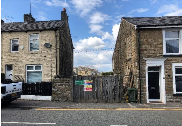
South east (front) elevation to Rosegrove Lane
